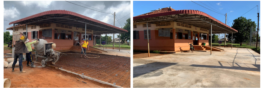
Improvement work at Bousra Public Health Centre - December 2019
